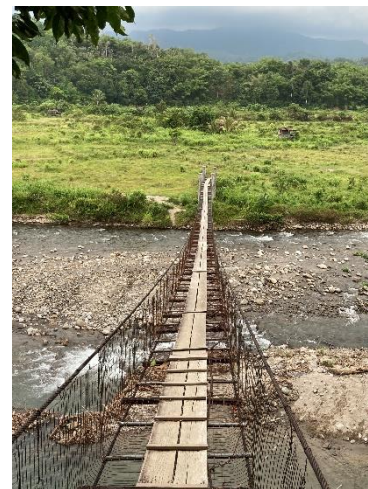
River crossing to W11
